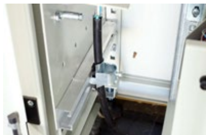
Adjustable cable glands suitable for different cable diameters
